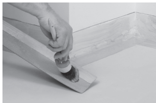
Apply glue on the floor and against the wall till the line.
